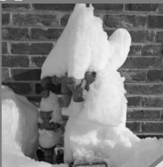
METER WITHOUT SNOW SHELTER
